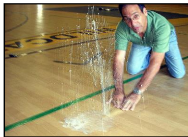
Photo from flooring failure in Bakersfield, CA.
