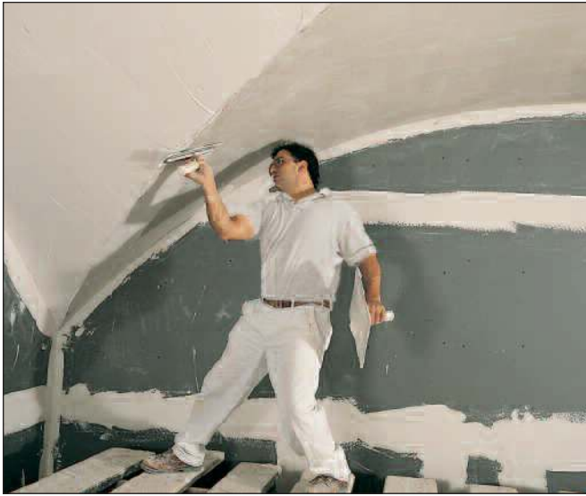
Design flexibility is achieved with veneer plaster systems.
