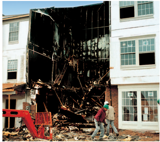
The fire-protection of gypsum-based Area Separation Fire Walls is demonstrated in dramatic fashion by the results of this actual townhouse fire in which the two-hour fire-rated assembly performed as expected in protecting adjacent properties. Break-away feature allowed collapse of fire-side structural framing without pulling down the entire wall.
