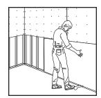
Hold the lower sidewall panel snugly against upper panel. A panel lifter (as shown) will
