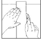
Using a straightedge and utility knife, score the drywall on the face paper side along the pencil line(s).
