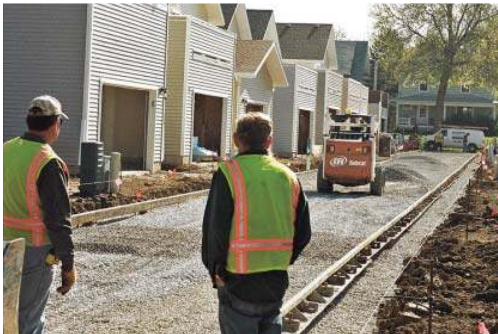
Figure 2. Pervious concrete requires a thick, well-drained gravel layer underneath, particularly in colder climates where trapped water can freeze and crack even the sturdiest pavement.
