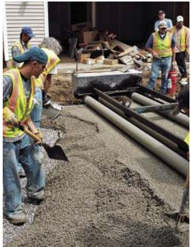
Figure 4. Fresh pervious concrete is dry and stiff, and requires plenty of manpower to place (above). A vibratory screed followed by a roller consolidates the mix (right). No floating, troweling, edging, or control joints are necessary (unless wanted for aesthetic reasons), which helps offset the higher costs for labor and subgrade prep.
