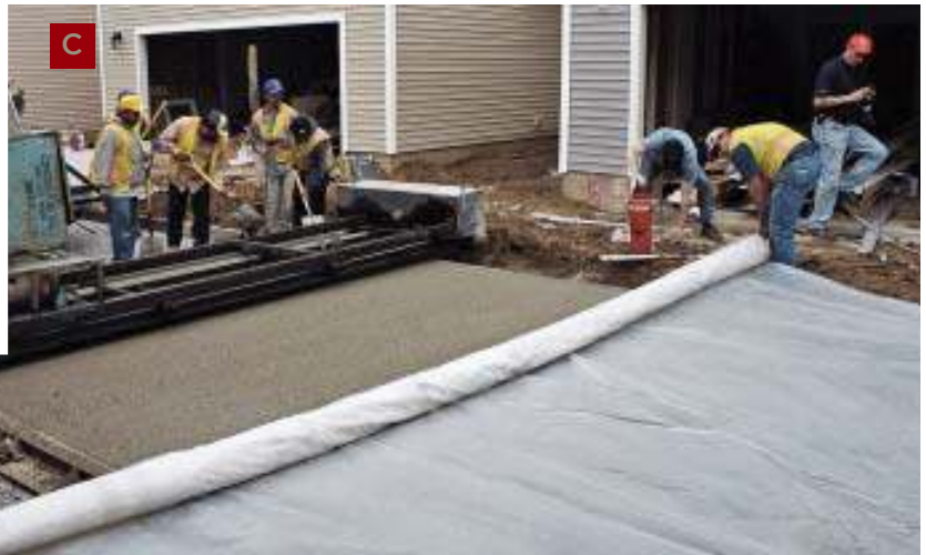
Figure 5. To slow hydration, newly placed pervious concrete is sprayed with a soybean-based curing compound (A, B), then quickly covered with polyethylene sheeting (C). The sheeting is weighted down with sandbags and left in place for seven days (D), and the paving is allowed to fully cure for 21 days before being opened up to vehicle traffic.
