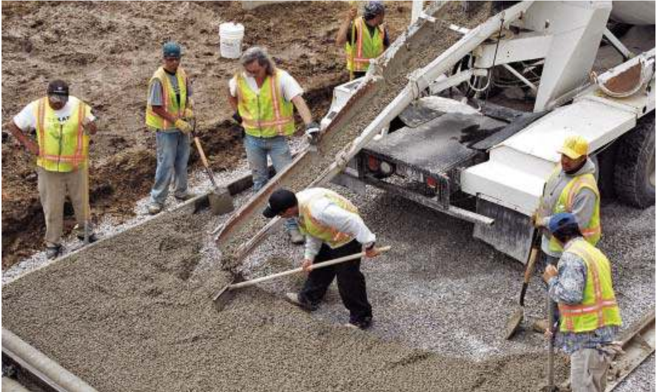
Figure 4. Fresh pervious concrete is dry and stiff, and requires plenty of manpower to place (above). A vibratory screed followed by a roller consolidates the mix (right). No floating, troweling, edging, or control joints are necessary (unless wanted for aesthetic reasons), which helps offset the higher costs for labor and subgrade prep.
