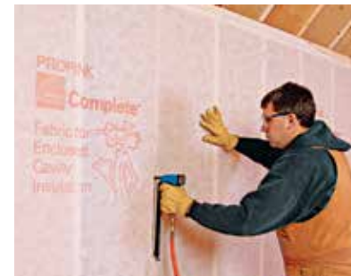
Fabric staples to studs quickly.
