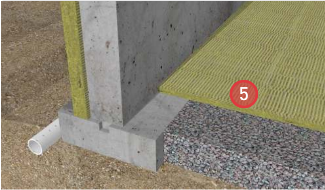
5. Install ROXUL® rigid board insulation at grade. Ensure the insulation is installed tight to the foundation wall.
