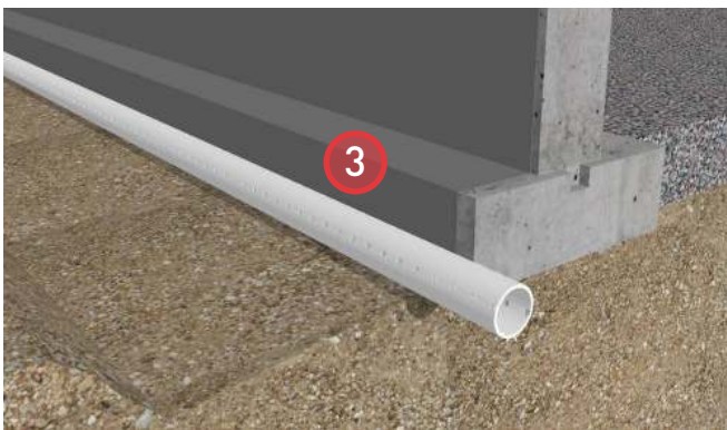
3. Install perforated pipe with filter fabric at the base of the footing and fill around with drain rock.
