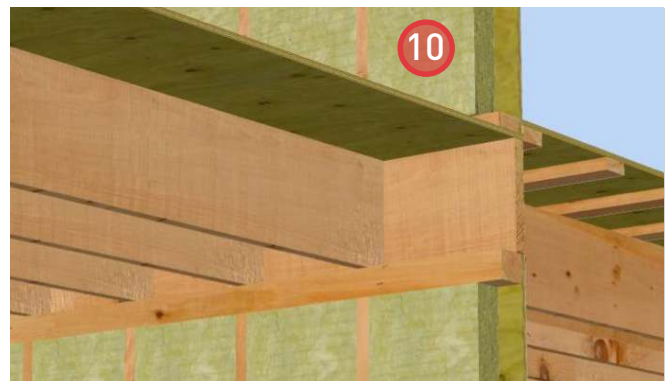
10. Install ROXUL® COMFORTBATT® in the interior stud cavities.
