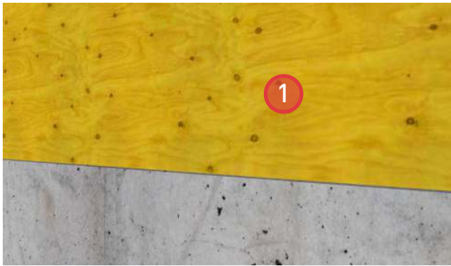
1. Typical wood frame construction at sheathing installation.
