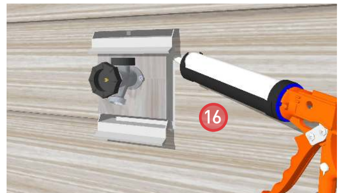
16. Apply sealant around the perimeter of the face plate and sill flashing (bottom and sides).
