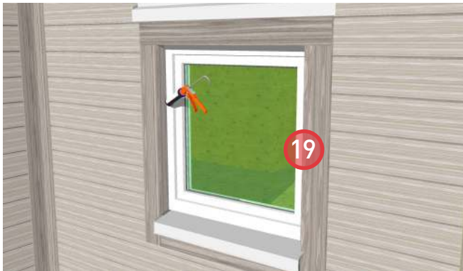
19. Install sealant around the perimeter of the window between the trim boards and the window frame (top and sides).
