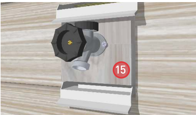
15. Install the cladding.
