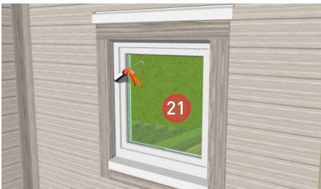
21. Apply sealant around the perimeter of the window (top and sides) between the frame and the window trim boards.
