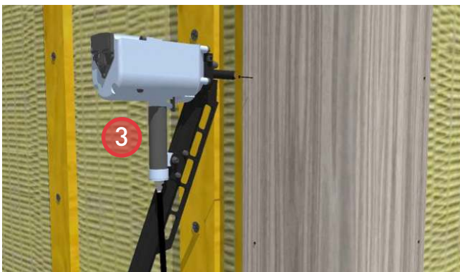
3. Install strapping as required to support the corner trim boards and cladding. Install corner trim boards.
