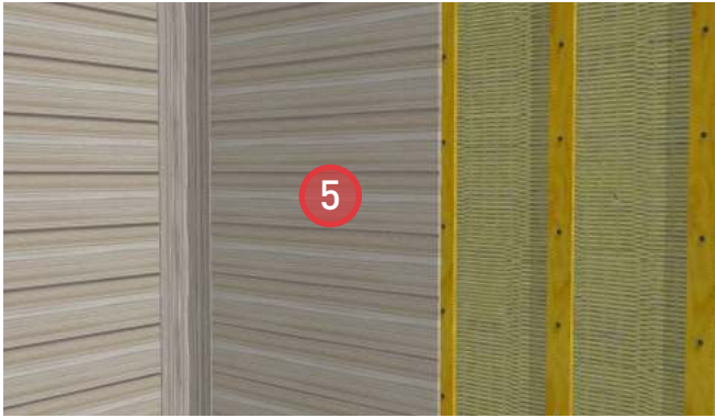
5. Install cladding.
