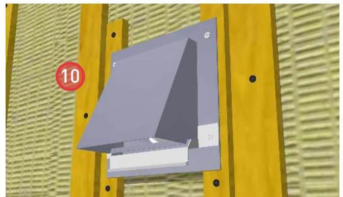
10. Install prefinished metal flashing below the exhaust vent hood.
