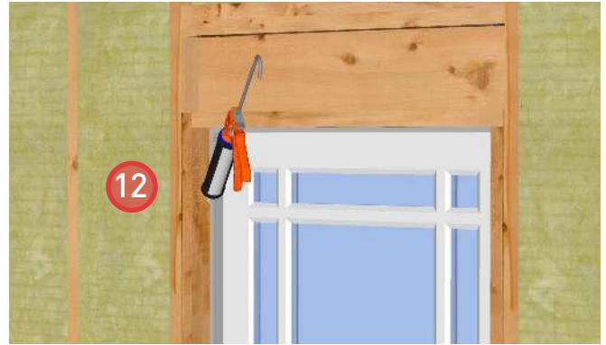
12. Install backer rod and sealant around the interior perimeter of the door frame to maintain air barrier continuity.
