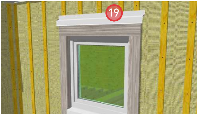
19. Install metal flashing to the strapping over the top window trim board.
