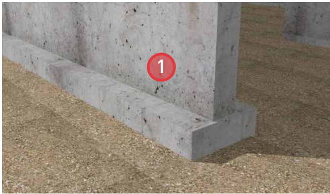
1. Intersection of the concrete foundation wall with the footing.
