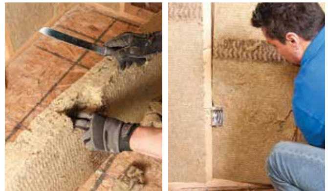
ROXUL COMFORTBATT® higher density batts make it simple for precise cutting to ensure a fit without gaps and voids.
