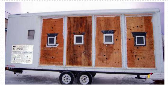
Exterior of the Mobile Test Lab at the end of the 2-year study, with the siding and insulation removed.
