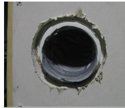
Figure 21: Install the gypsum
