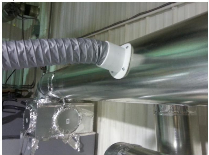
Figure 19: Screw the saddle on the trunk
