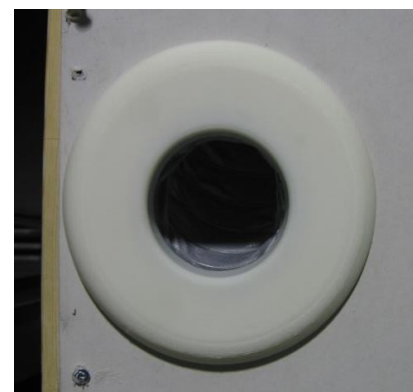
Figure 22: Screw the diffuser on the collar
