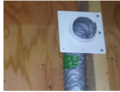
Figure 20: Attach the collar on the wall stud
