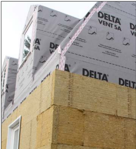
Figure 7: Using DELTA®-VENT SA membrane as an air barrier with mineral fiber insulation as vapor permeable continuous exterior insulation prevents condensation from air leakage and vapor diffusion, especially in cold climates.
