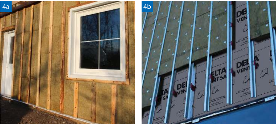
Figure 4: (a) Wood furring strips installed with screws for attachment of cladding over DELTA®-VENT SA (Refer to Detail 04 and Detail 06) and (b) Cascadia Clips® installed over DELTA®-VENT SA.
