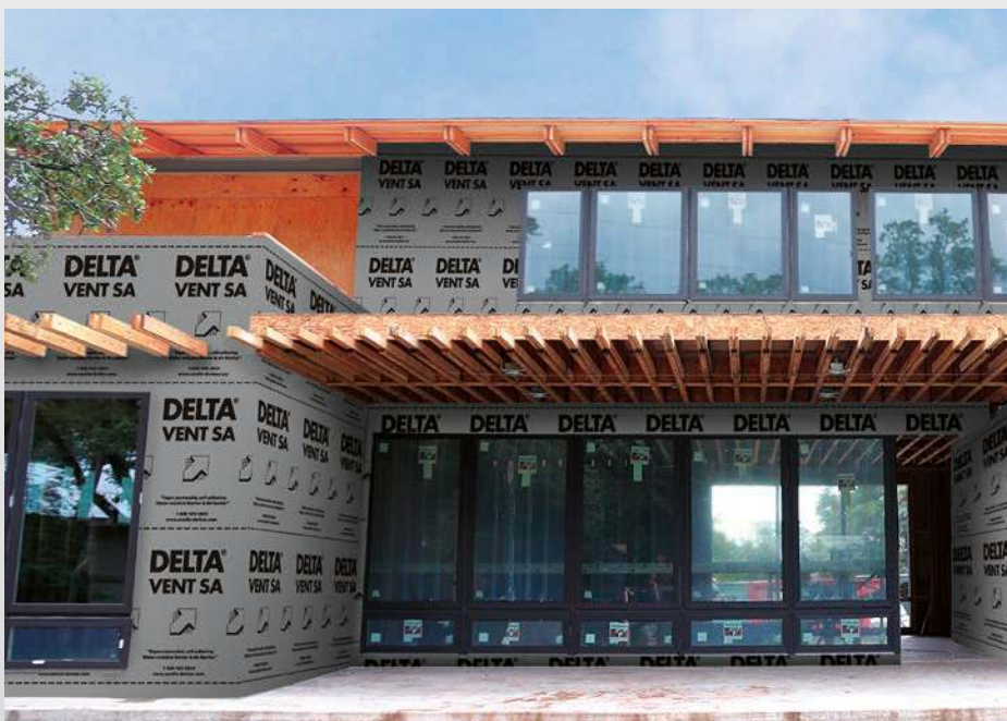
Air barrier application in residential construction
