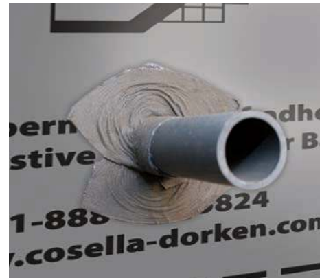
Air barrier continuity at penetrations
