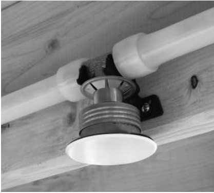
Figure 1-2: ProPEX tee with concealed sprinkler head
