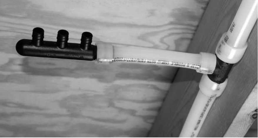
Figure 7-1: Feed plumbing fixtures via EP multiport tees
