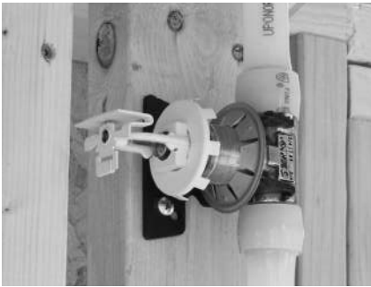
Figure 1-3: ProPEX tee with horizontal sidewall sprinkler
