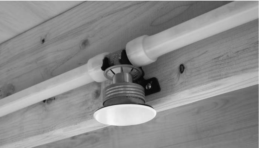
Figure 7-2: Uponor LF brass fire sprinkler adapters
