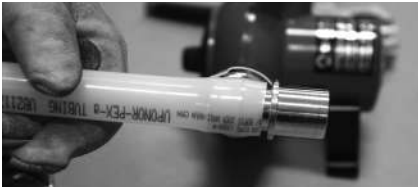
Figure 6-14: Gently heat tubing
