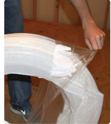
2. Using an Uponor-approved safety cutter (see page 2 ), remove the outer clear plastic layer. Note: Do not remove the inner white plastic layer.
