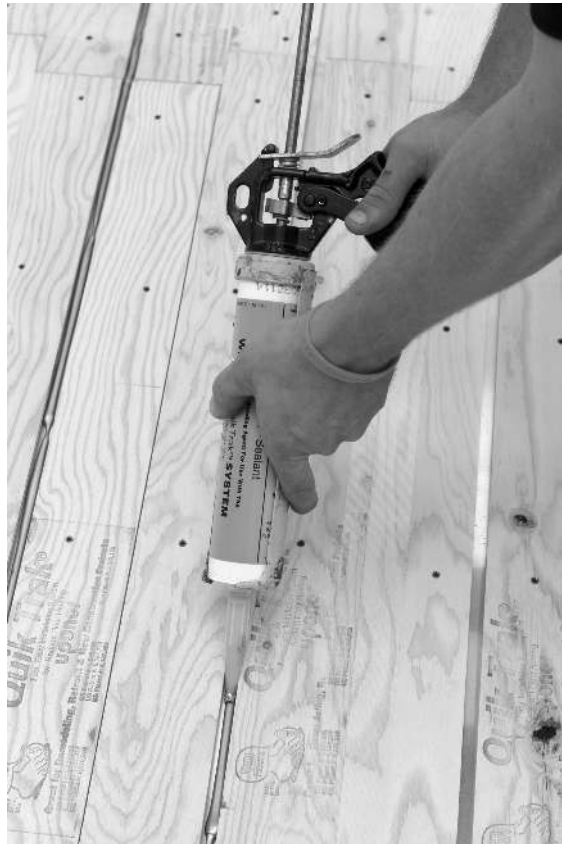
Figure 28: Apply a thin, \frac{1}{8} " bead of 100% silicone sealant to the entire length of the Quik Trak straight panel grooves. Do not apply the silicone sealant to the return panel grooves.
