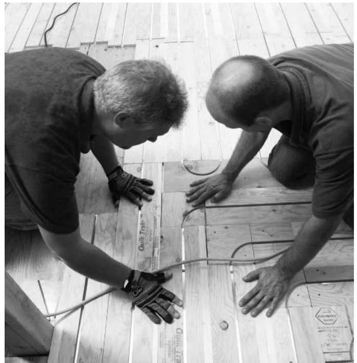
Figure 4: Installing Quik Trak straight panels
