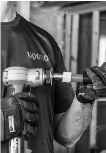
Figure 3-5: Making a ProPEX connection
