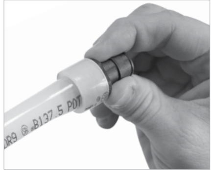
Figure 3-12: Insert the fitting
