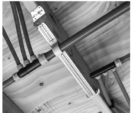
Figure 5-9: Multiport tee installation
