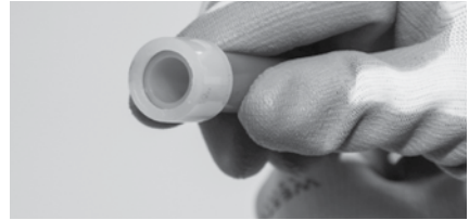
Figure 3-8: Ensure pipe reaches ring's stop edge
