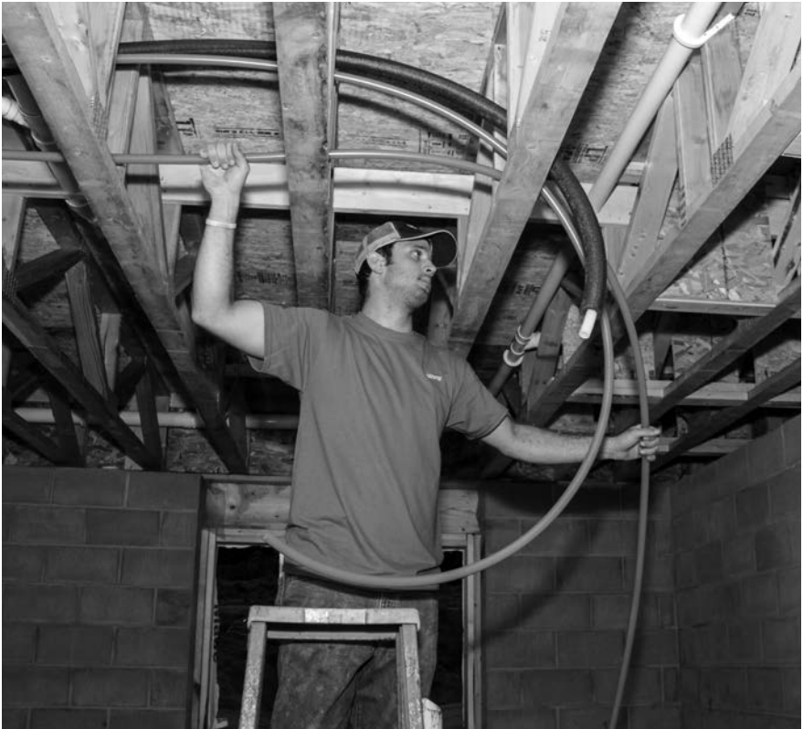
Figure 5-1: Running Uponor AquaPEX main lines through open-web trusses
