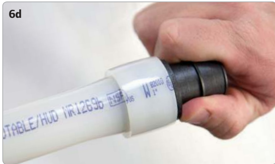
Insert ProPEX Fitting into 1" Uponor PEX-a Piping.
