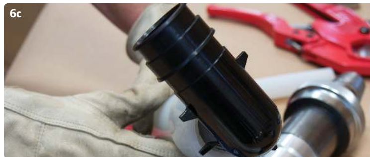
Insert ProPEX Fitting into 2" Uponor PEX-a Piping.
