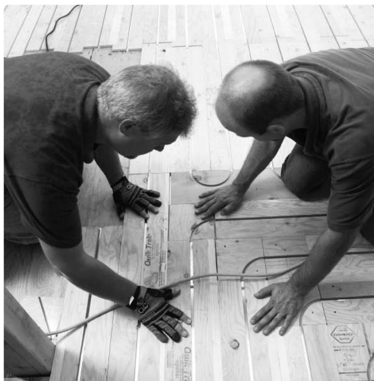
Figure 4: Installing Quik Trak Panels
