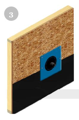
Slide the weather resistant barrier underneath the Quickflash® panel to the bottom of the pipe.
