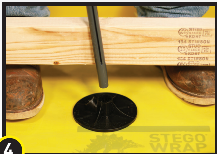
1 Ensure the press-fit center hub of Beast Foot is positioned in line with the form to be set. (Tip: pulling a string line or snapping a chalk line can be a helpful aid).
