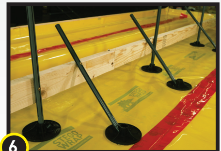
3 Apply downward pressure for 5 to 10 seconds; Beast Foot's engineered adhesive is pressure sensitive. (Tip: In cold weather, extra time may be needed while applying pressure).
