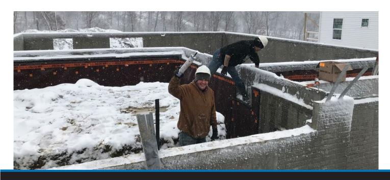
When protecting foundations, the feasibility of applying wall waterproofing below temperatures of 40°F (4°C) is a common question. Particular products require above-freezing temperatures to be applied. If a fluid-applied product is selected for installation during lower seasonal temperatures, the field applicator may face some of the following issues, compromising the integrity of the liquid membrane:
