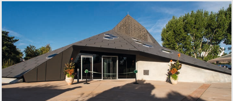
Unique approach to main entrance
