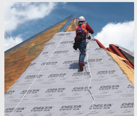
DELTA®-VENT SA adhered to plywood
