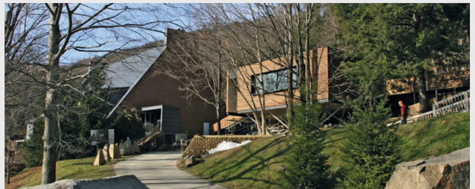
Tranquil approach to main entrance
