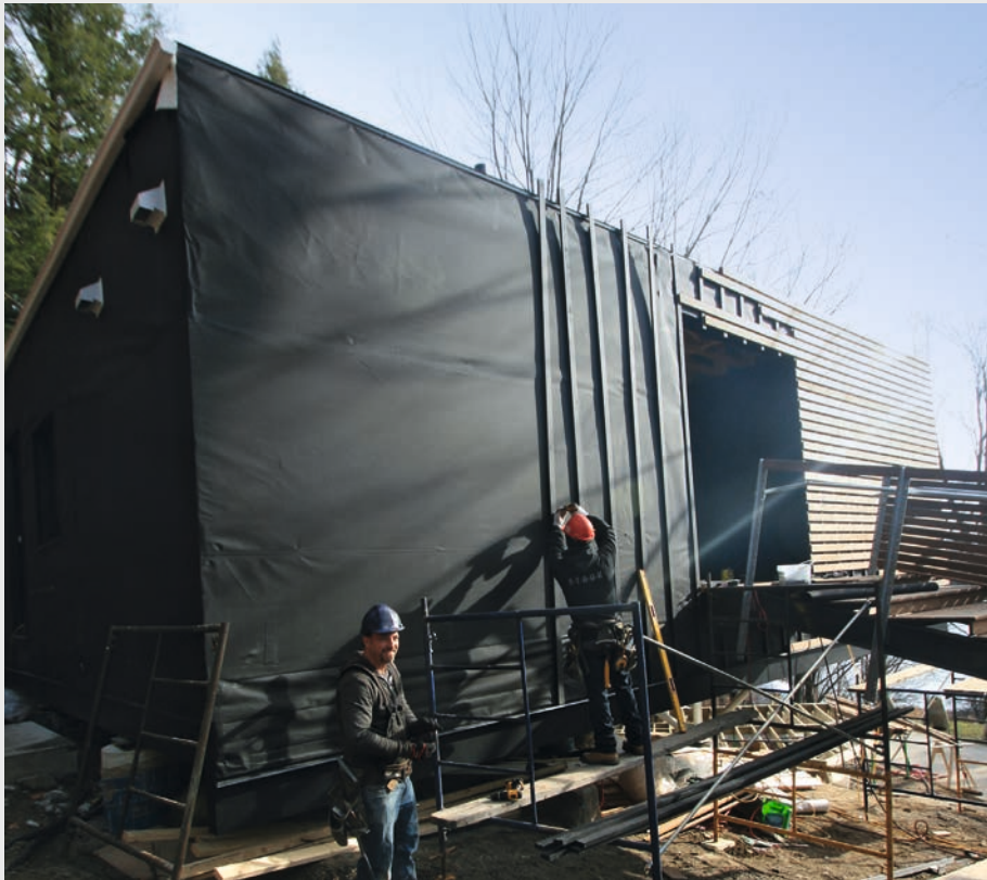
Installation of cedar furring strips over DELTA®-FASSADE S
