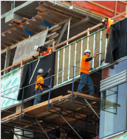
DELTA®-FASSADE S is rolled into place for a trouble-free installation.
