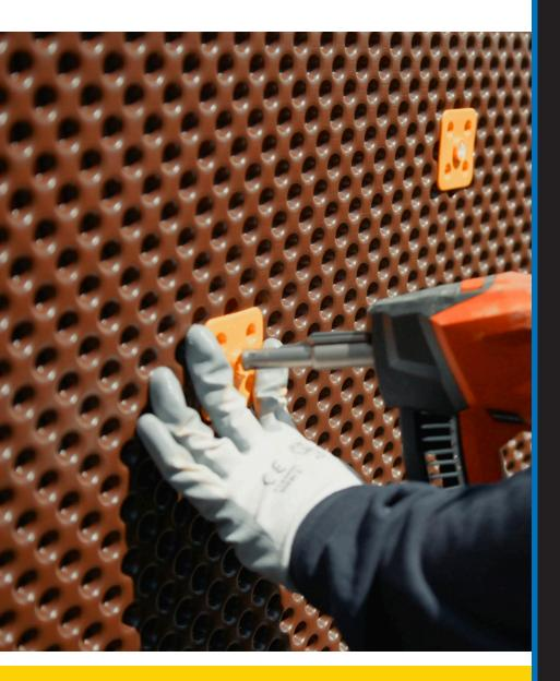
HOLDING POWER DELTA®-FAST'ner 0.95 kN / anchor DELTA®-PLUG 0.54 kN / anchor Plastic Washers 0.39 kN / anchor
