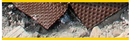
Cut membrane at corners from the outside edge of the footer to wall footer junction
