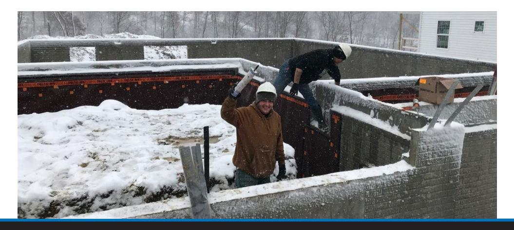
When protecting foundations, the feasibility of applying wall waterproofing below temperatures of 40°F (4°C) is a common question. Particular products require above-freezing temperatures to be applied. If a fluid-applied product is selected for installation during lower seasonal temperatures, the field applicator may face some of the following issues, compromising the integrity of the liquid membrane:
