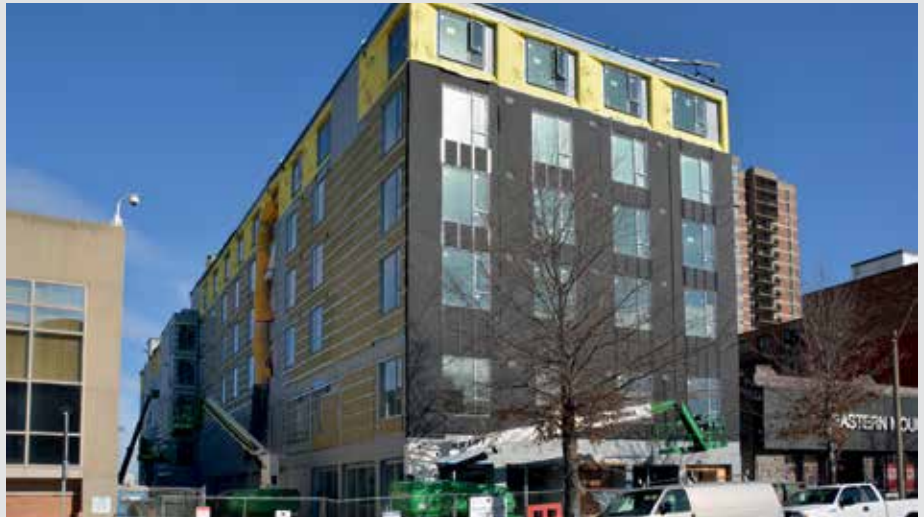
DELTA®-FASSADE S is designed specifically for the demands of open-joint cladding
