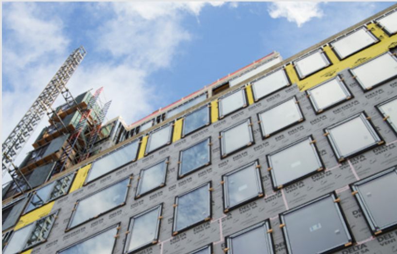
24 2 nd Avenue needed an advanced weather-resistive barrier that contributes to a high-performing, energy-efficient building
