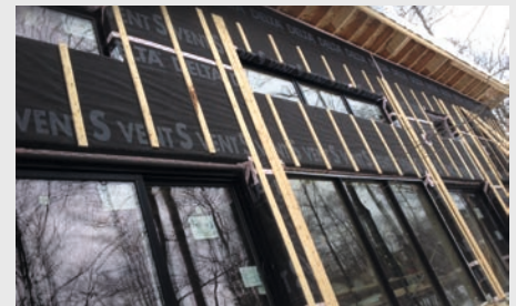
DELTA®-VENT S was used as a secondary air barrier providing additional air tightness.
