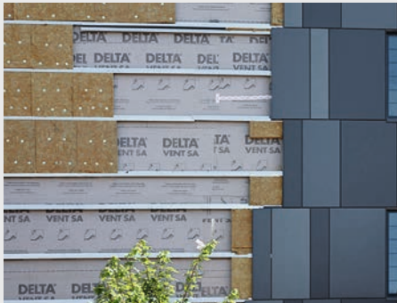
Installation of rainscreen cladding
