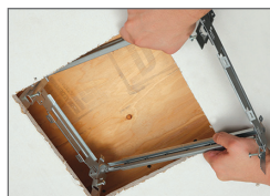
Insert single-hinged Flex-Z Fast® installation bracket
